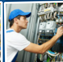
Technician (equipment maintainers)
